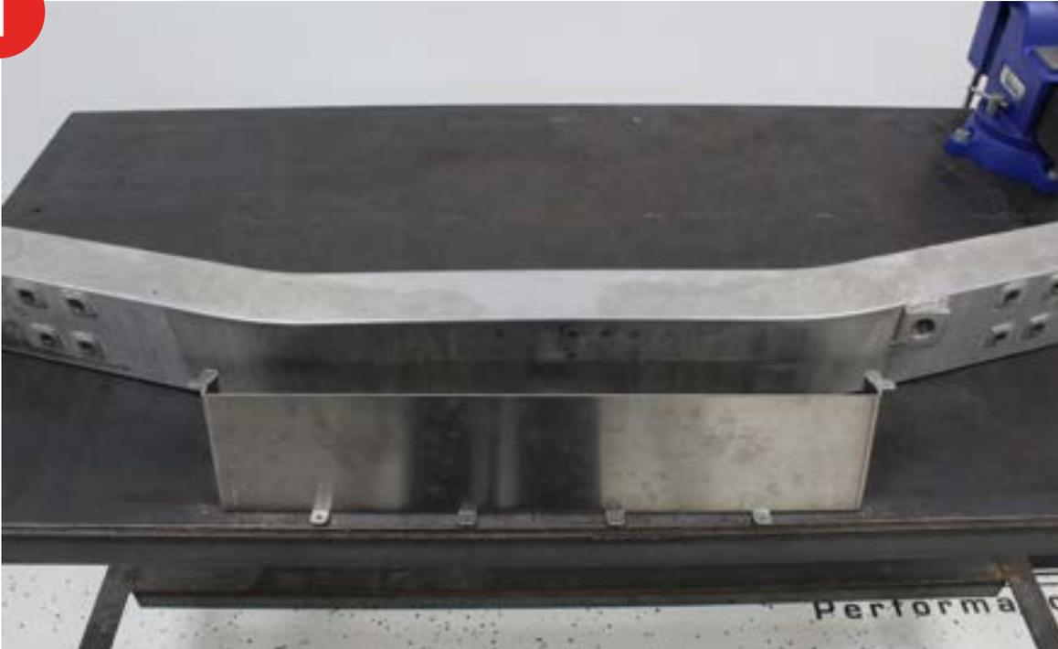
2. Start by placing the patch panel over the rear of the crash beam and marking it. Make sure it is centered on the beam.
